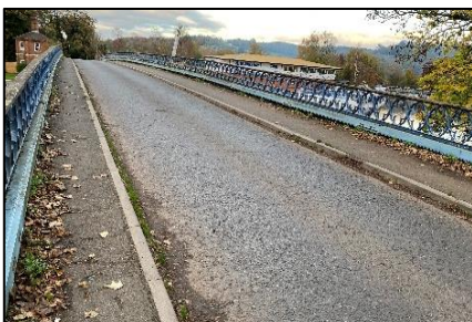
Left Cookham Bridge looking north.
