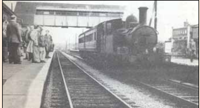
Cookham's railway station originally had a main track, passing loop and pedestrian footbridge as seen above.
