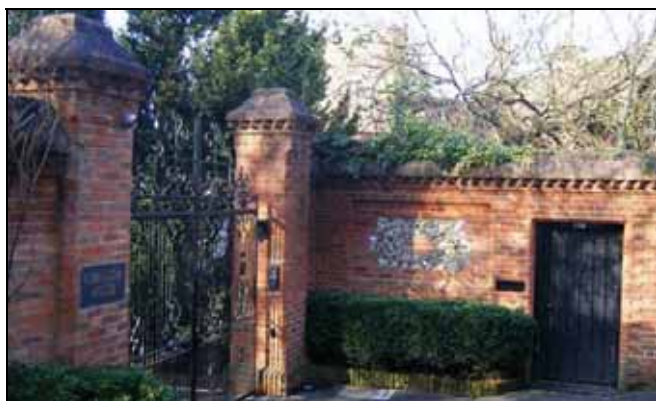
A recent extension to a striking decorative wall in Gibraltar Lane links to the gateway (left), very successfully matching the original wall (left again). The extended section is further enhanced by a reclaimed historic door.
