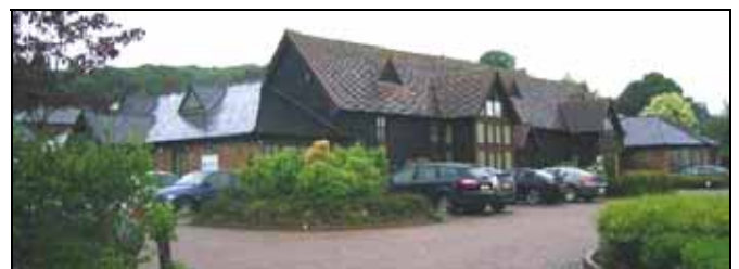
The Courtyard Barns on Choke Lane, sensitively converted into business premises.
