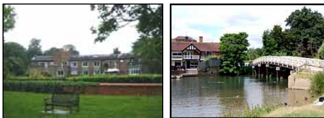
Above left: The Riverside Nursing Home, overlooking Bellrope Meadow and the Thames. Above right: On Lulle Brook is the unspoilt façade of Lullebrook Manor.
