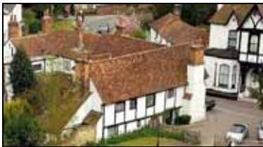
Red roofs of Cookham: clay tiles are prominent throughout the three settlements, although slate dominates in certain areas.
