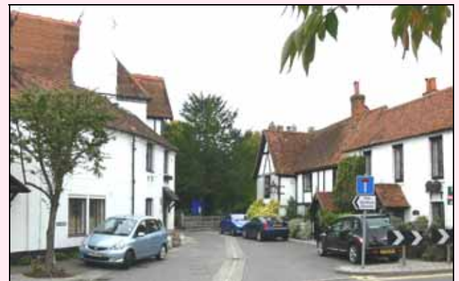
Above: Church Gate precinct with Churchgate House at centre right.
