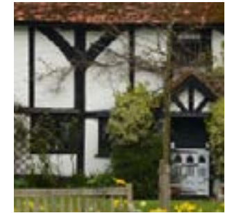
Exposed timber framing
