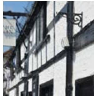
Exposed timber framing
