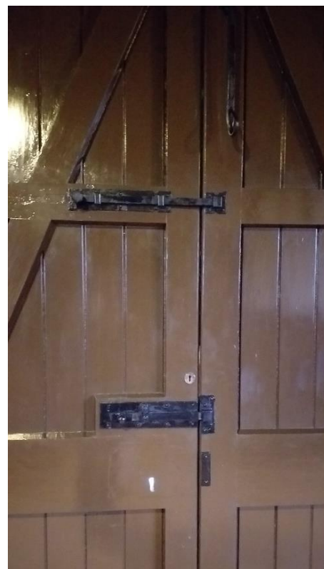
Large door, nearest the road, showing the bolts at the top and across the door.
