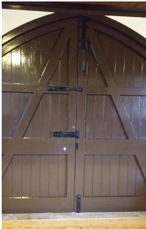
Large door, nearest the road, showing the bolts at the top and across the door.
